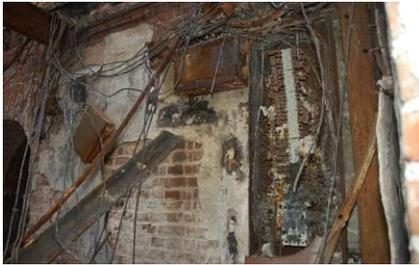
We now know the cause of the fire. In November 2015 the official report from the South East Fire Investigation Group was published. The conclusion was that the fire was accidental, caused by an electrical fault in a distribution board located in the basement. The fire could not be contained due to the nature of the building's construction and the lack of internal fire compartmentalisation. In December the
